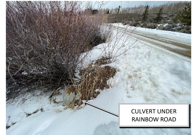
PHOTO OF CULVERT
